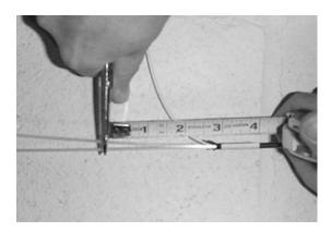
Figure 7 – Cut the strength members at the required length.
