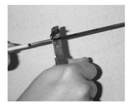
Figure 3 – Shave the cable jacket on top of the strength members.
