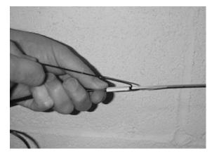
Figure 6 – Removing the outer cable jacket.
