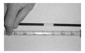
Figure 2 – Mark the jacket removal length.
